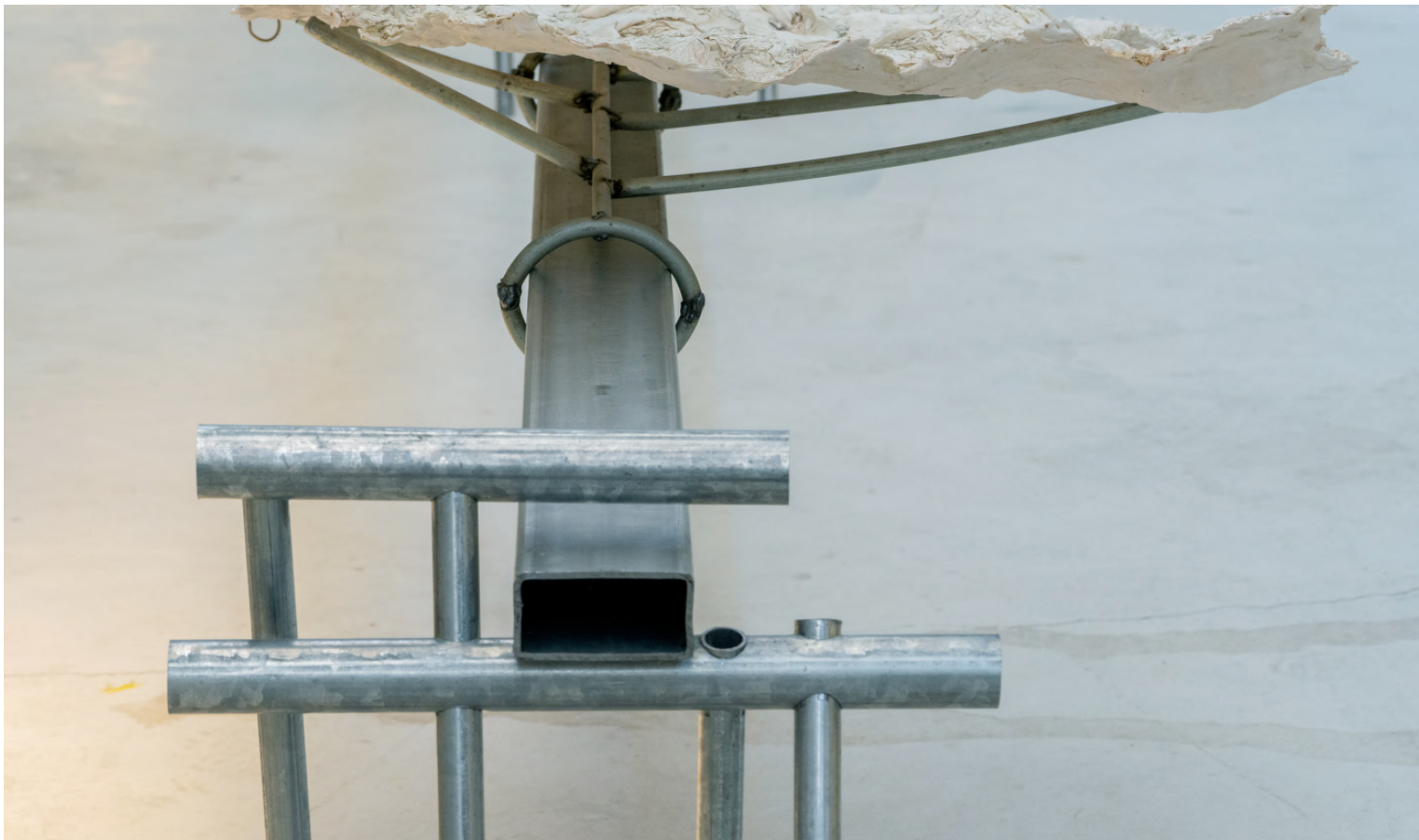
Galvanized iron pipe legs connected by pressure, Galvanized iron profile and welded Galvanized iron rib seatings
